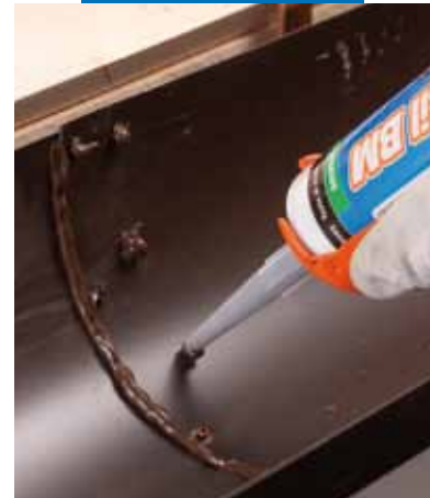
Sealing the heads of rivets
